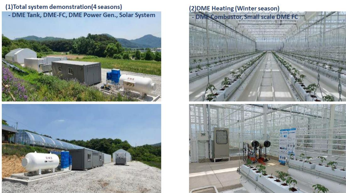
Figure 35: Installation of “DME-H2 FC System” and “DME Power Gen.” by Bio Friends (Cho, DME, rDME and H2 Business in Korea, 2022)
